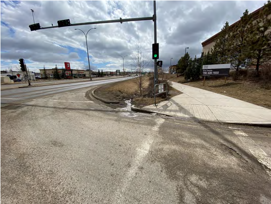
The southwest corner of Southridge Drive and Westmount Road where people walking / rolling are not permitted to cross using the south leg and where there is no existing curb ramp at the corner.
