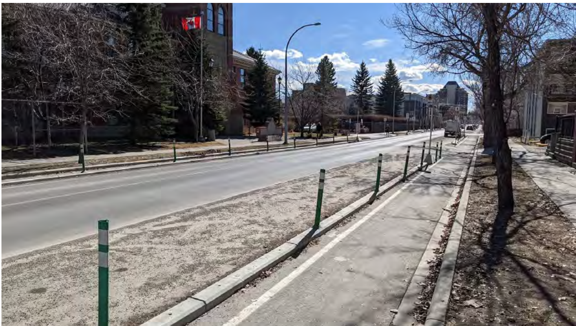
Examples of quick-build cycling facilities in Calgary. Top photo shows a neighbourhood bikeway with diverters and temporary traffic calming curbs to prioritize the road for people cycling. Bottom photo shows a protected bike lane with quick build materials including delineator posts and precast concrete curbs.
