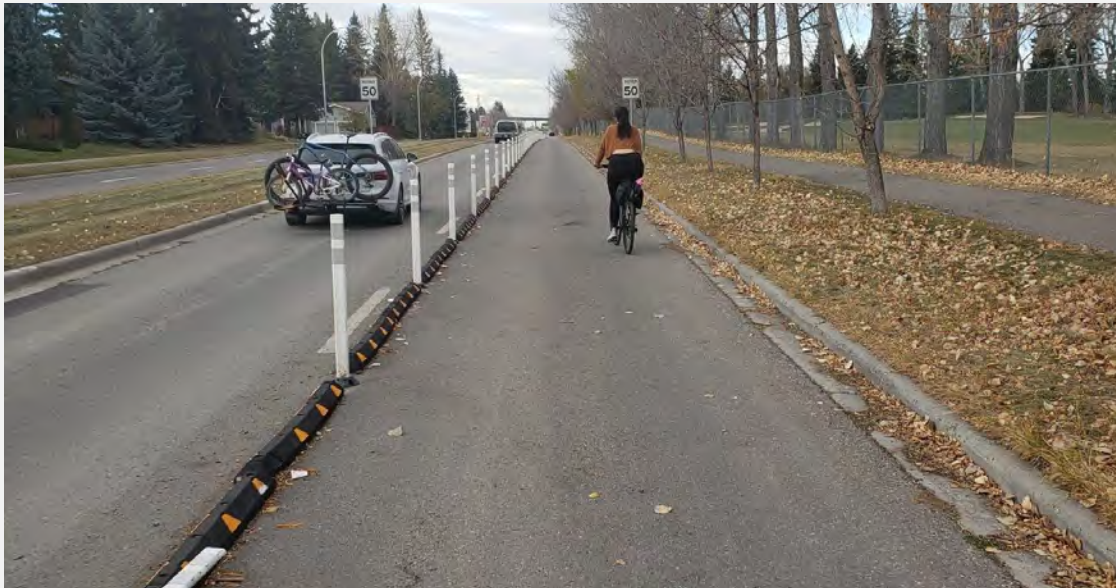
Example of a protected bike lane in Calgary, AB using rubber curbs and flexible delineators. Credit: Bike Calgary.
